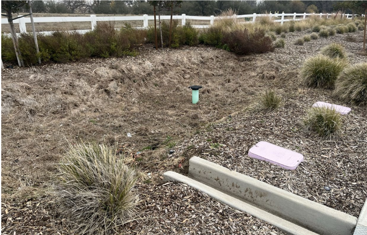
Photo No. 13 Small stormwater infiltration basin in southeastern portion of Lot C-43
