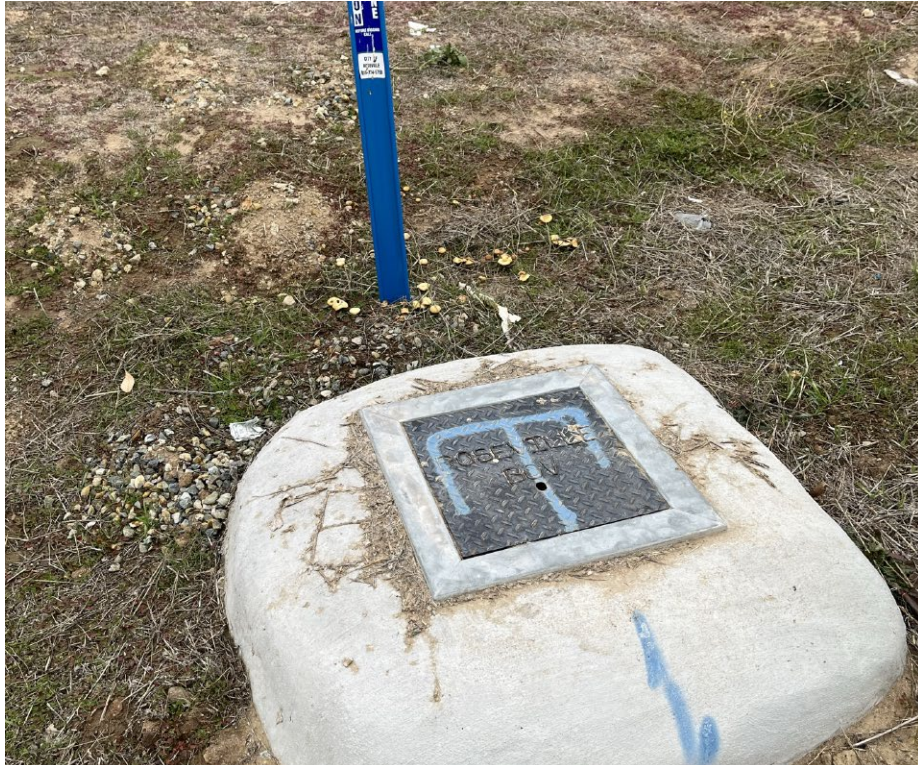
Photo No. 9 Water pipeline blowoff valve in southeastern portion of Lot C-43
