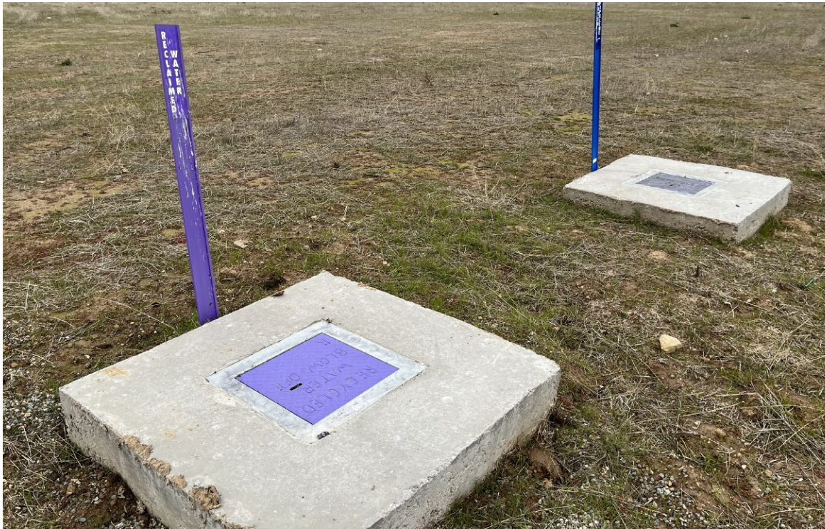
Photo No. 11 Water pipeline and recycled water blow off valves in northwestern portion of Lot C-43
